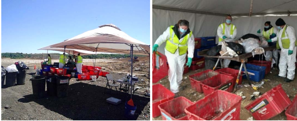
Figure 2-6 Sorting Work Area
